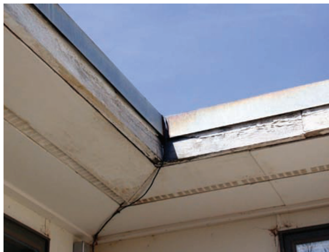
Openings under roof line
